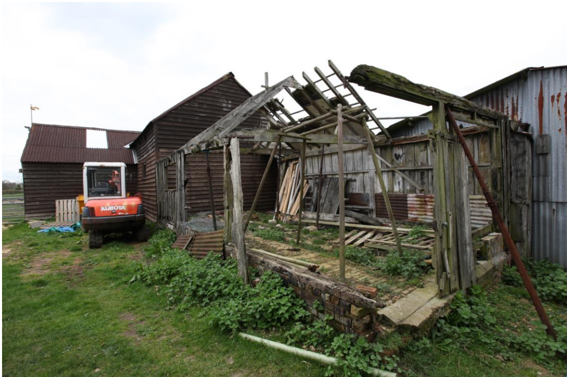
Illus. 6 The exterior of the partly dismantled southern shed (4) from the south-west showing its post-and-rail wall fabric with the barn (1) to the left and the corrugated iron southern yard shed (5) to the right.
