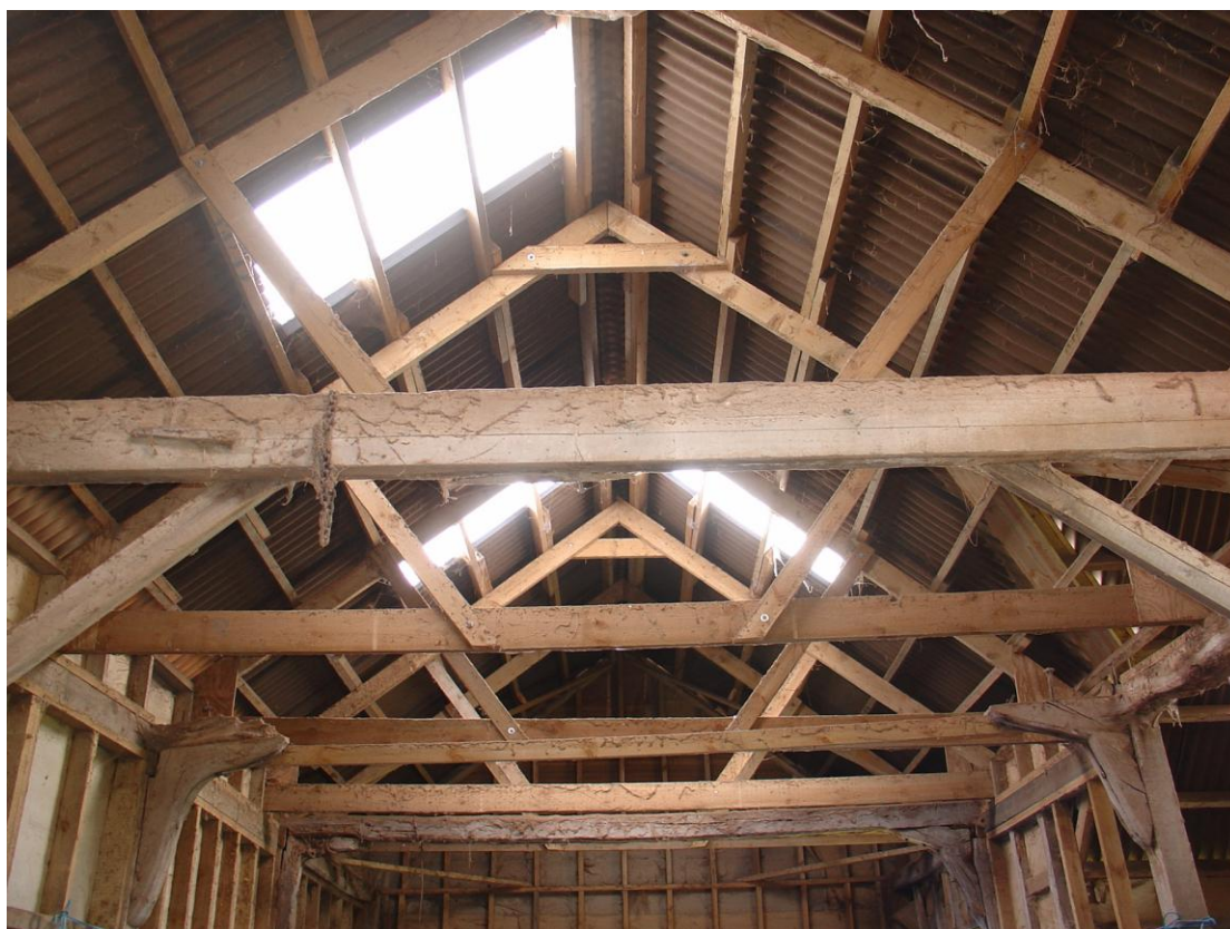
Illus. 3 2006 old photograph. The interior of the barn (1) from the north showing the largely 20 th century softwood timber of its walls and roof (all hidden by boarding at the time of inspection)
