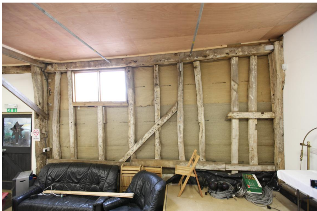
Illus. 10 The western interior of the barn's northern bay (1a) showing empty trenches for a missing wall brace to the right and later framing with a diagonal primary brace in the style of the 18 th and 19 th centuries to the left.
