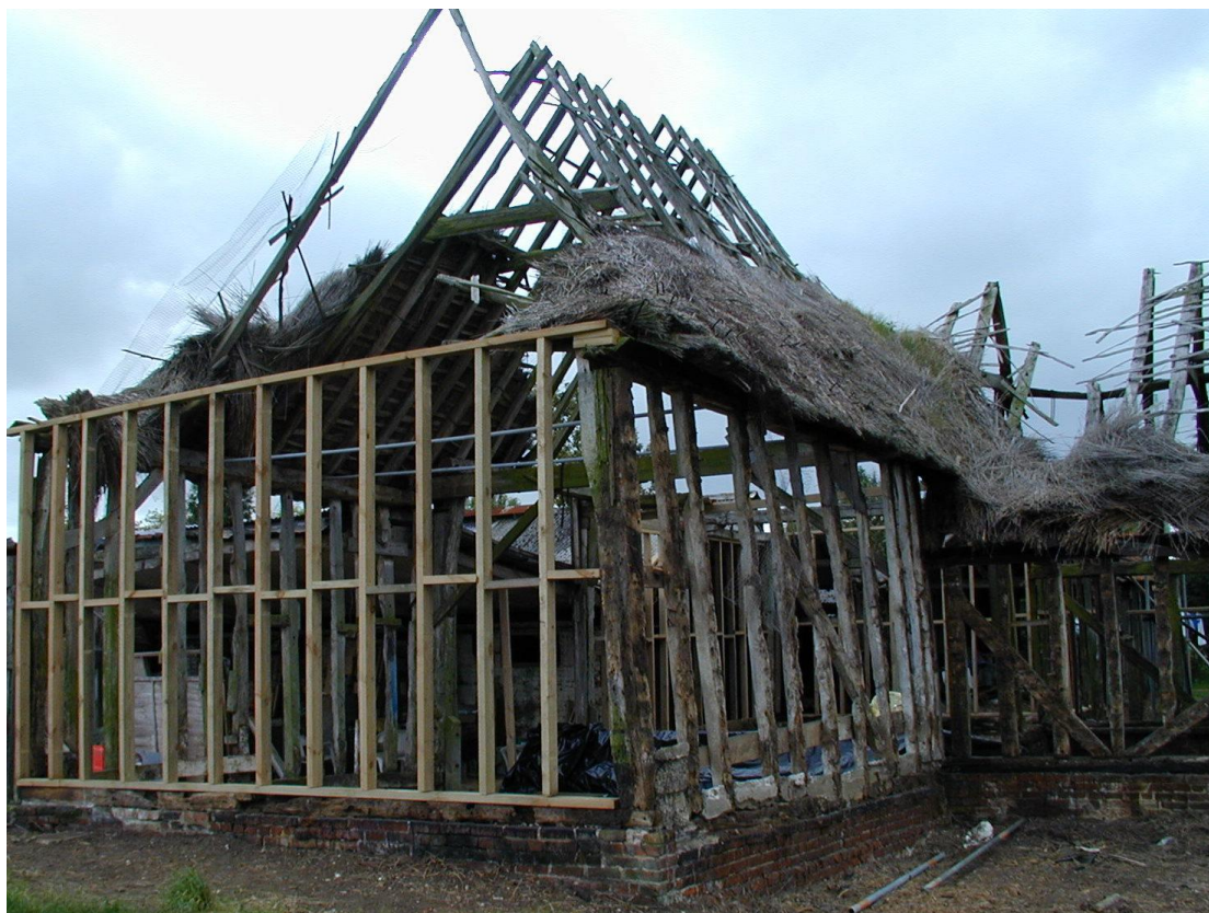
Illus. 2 Circa 1990s old photograph. The exterior of the barn (1) from the north-west during storm repairs showing the remains of its original thatched clasp-purlin roof.
