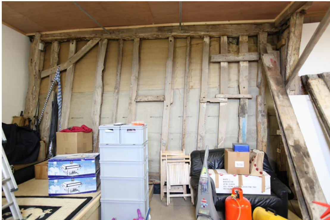
Illus. 9 The eastern interior of the barn's northern bay (1a) showing the intact early-17th century frame with original reverse-cranked trencled brace to left. A number of additional studs have been inserted between the original timbers.
