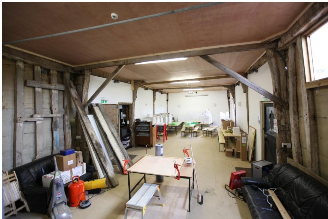
Illus. 8 The interior of the barn (1) from the north showing the recent wallboard and ceiling board which conceals most of the timber structure.
